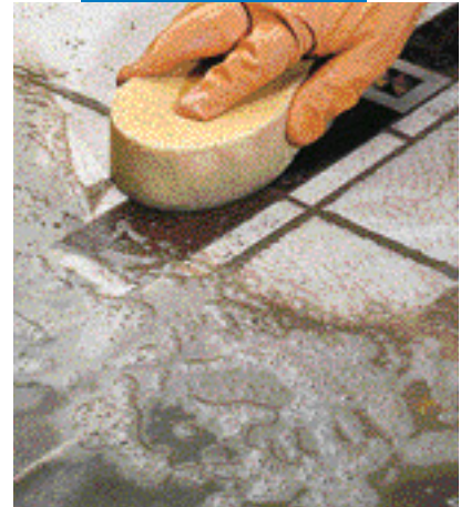
Finishing a ceramic tile floor with wood inlays with a sponge
