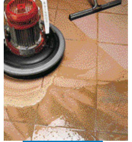
Finishing a porcelain tiled floor with single-brushed power float or rubber squeegee
