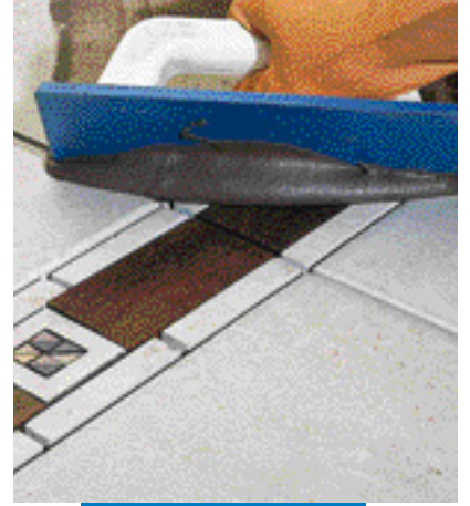
Grouting a ceramic tile floor with wood inlays with a trowel
